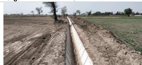
Picture 3.4: A view of Lined Portion of Watercourse no 10666 R
