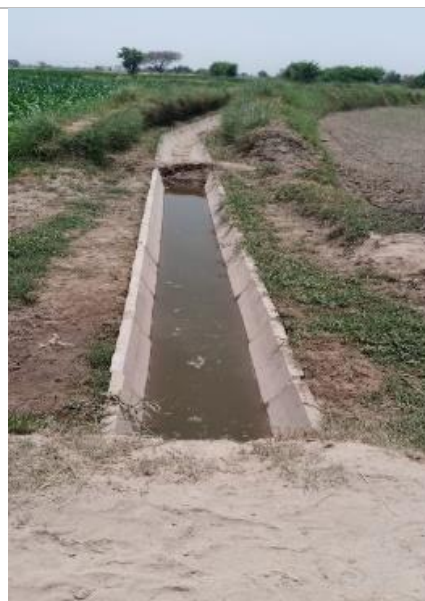
Picture 3.7: A view of lined portion of watercourse no. 26066/L
